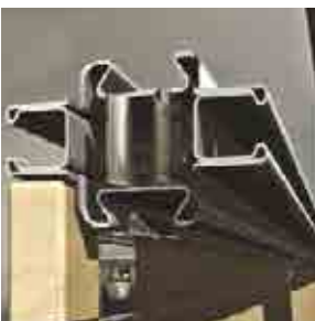
08 Simple clip are used to secure boards onto the metal frame.
