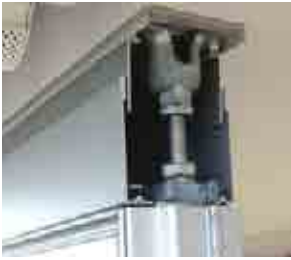
01 Ceiling & Integrated Floor Connection
